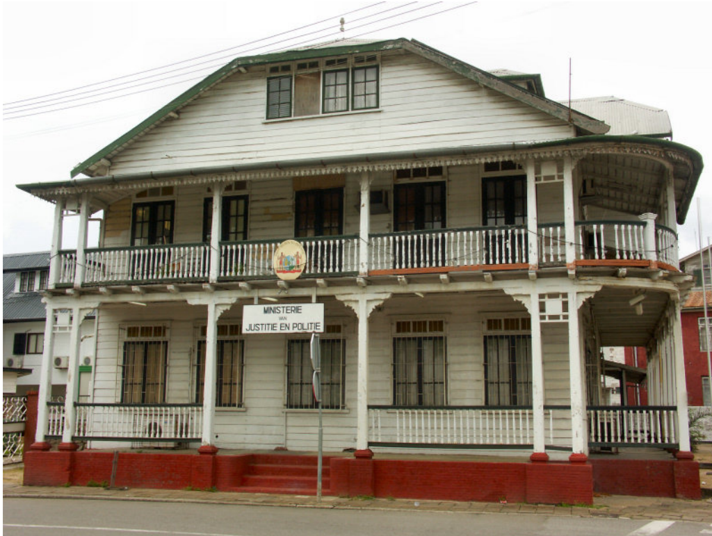
Figure 2: The Department of Justice and Police in Surinam, which is in bad condition
