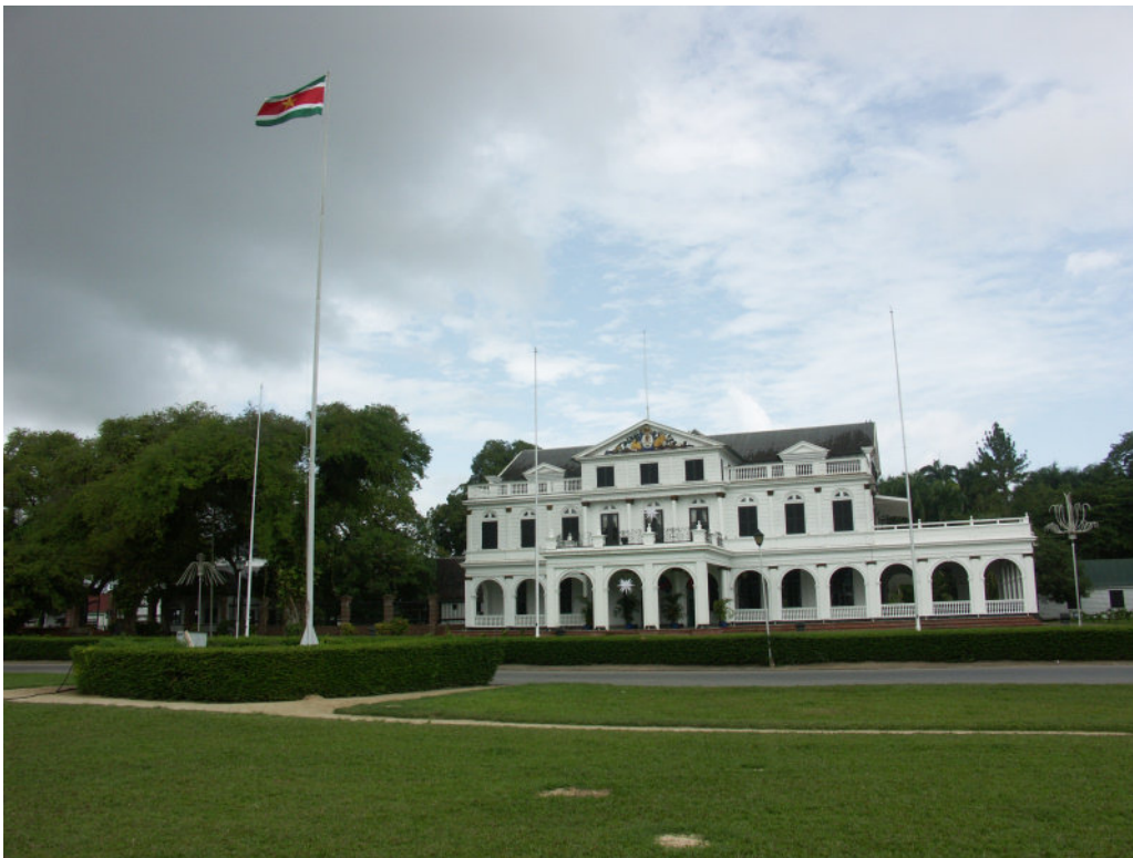
Figure 1: The Presidential Palace in Surinam, which is in fine condition
